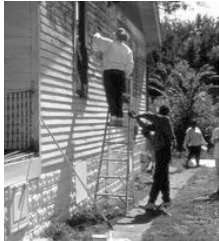
Paint-up, scrape-up work weekends
