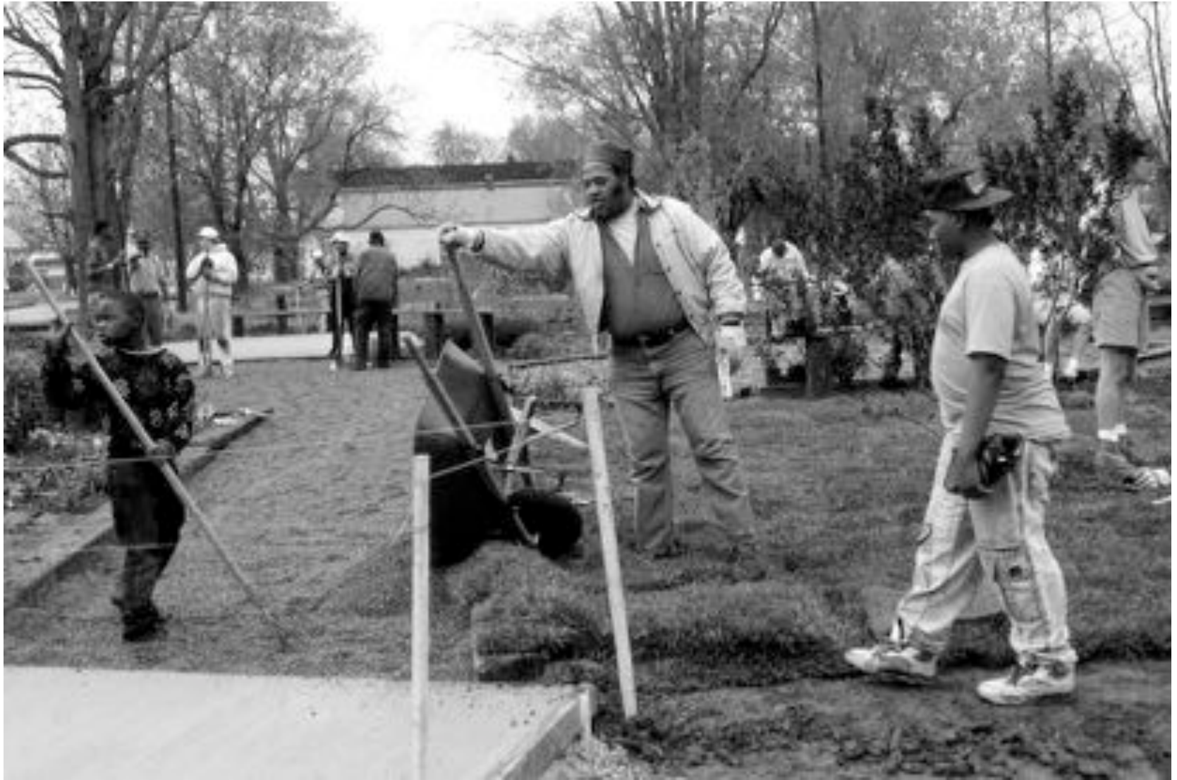
Construction of Illinois Avenue Playground
